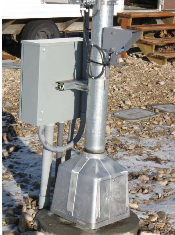
Figure 3.10: System 5 (Calonder Energy 1) (Photo: Marcel Huijser, WTI/MSU).
