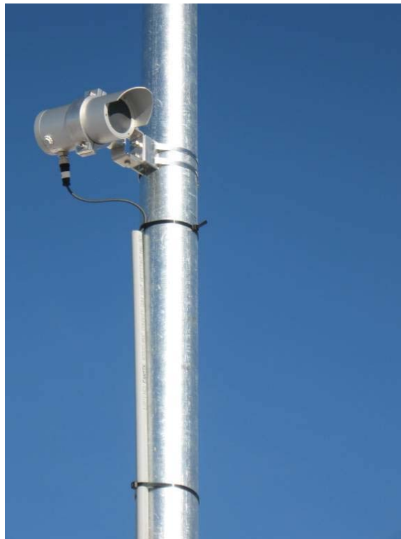
Figure 3.11: System 6 (Calonder Energy 2) (Photo: Marcel Huijser, WTI/MSU).
