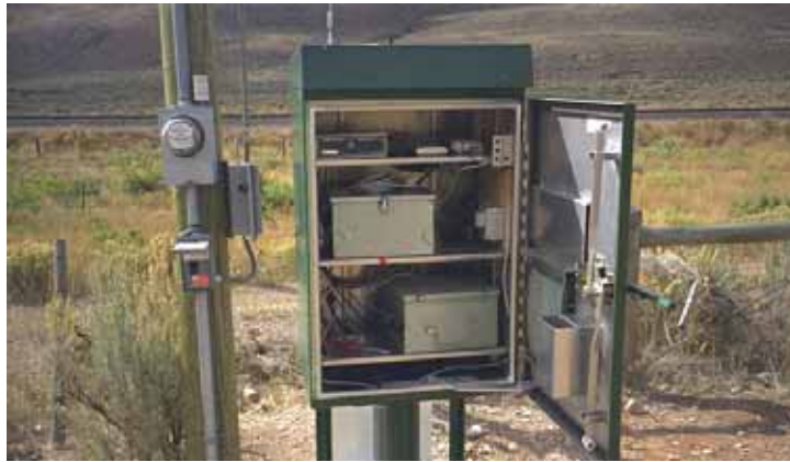
Figure 4.20: Control cabinet at Nugget Canyon, Wyoming, USA. The large boxes are the counters for the animal detections and traffic. The upper shelf holds equipment for downloading data. This equipment used AC power. (Photo: Matt Johnson, WYDOT)
