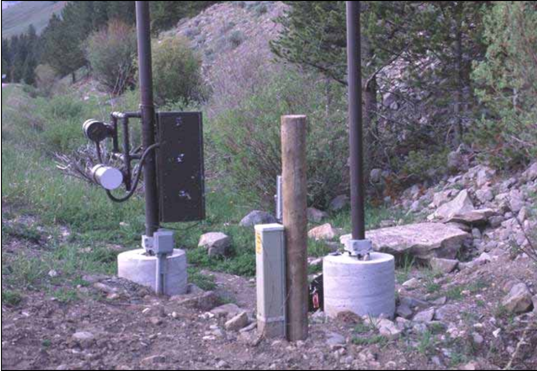
Figure 8.1: Some of the concrete foundations were in the clear zone and too high above the ground. This is the master station. The wooden post on the foreground is for the link to the land-based phone line. (Photo: Marcel Huijser, WTI-MSU)
