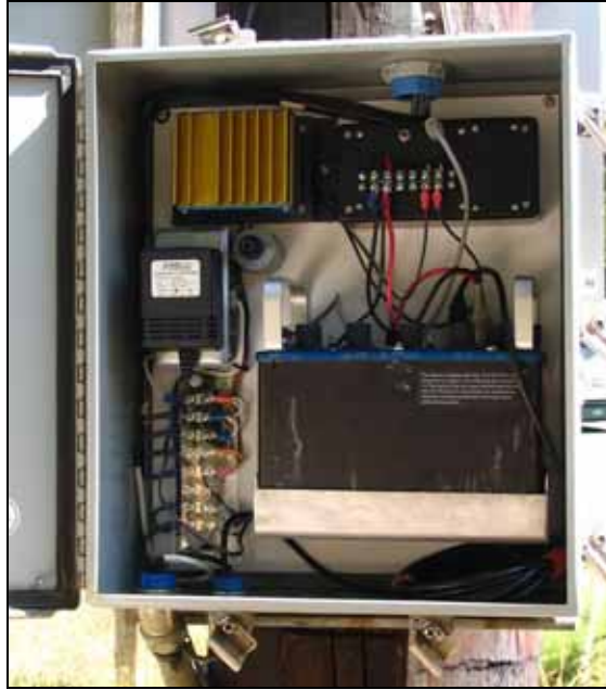
Figure 4.25: Cabinet with electronics for automated scanning for frequencies of radio collared elk and battery at one of the receiver stations in Sequim, Washington, USA (Photo: Marcel Huijser, WTI-MSU)
