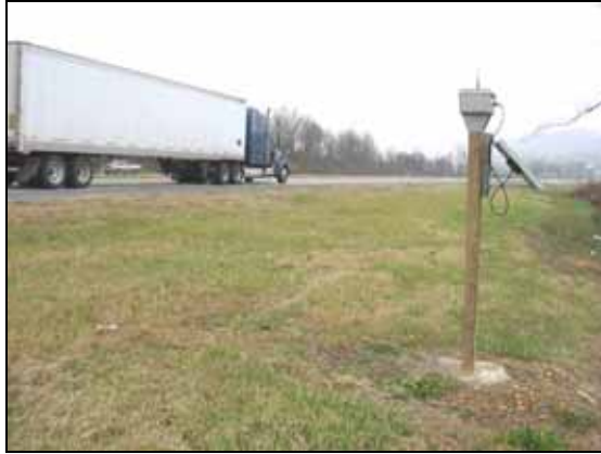
Figure 5.15: A station at the PA site. The sensors and battery are located inside the grey box on top of the pole. The solar panel is attached to the side of the pole. (Photo: Marcel Huijser, WTI-MSU)
