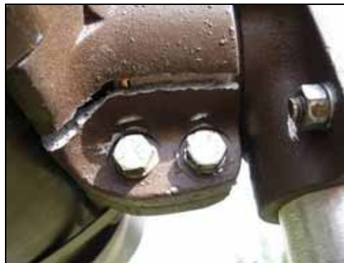
Figure 6.8: The brackets holding the sensors cracked as a result of extreme temperature fluctuations at the MT site (Photo: Marcel Huijser, WTI-MSU)
