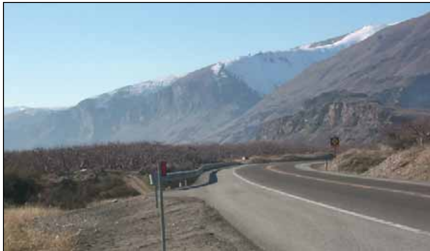
Figure 4.35: The area approaching the system in Wenatchee, Washington, USA (Photo: WSDOT, NorthCentral Region)
