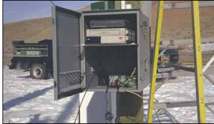
Figure 4.21: Video recorder system at Nugget Canyon, Wyoming, USA (Photo: Bill Gribble, WYDOT)
