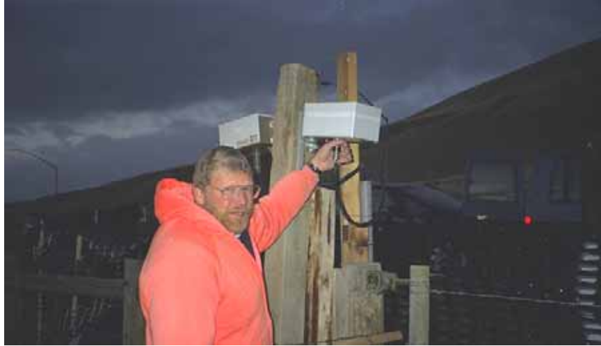
Figure 4.19: Microwave radar transmitters at Nugget Canyon, Wyoming, USA (Photo: Bill Moore, WYDOT)
