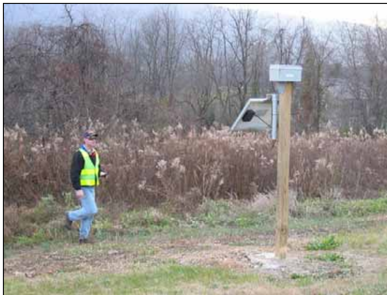
Figure 7.24: Jon Fleming (PennDOT) approaching one of the stations at the PA site to test the reliability of the system (Photo: Marcel Huijser, WTI-MSU)
