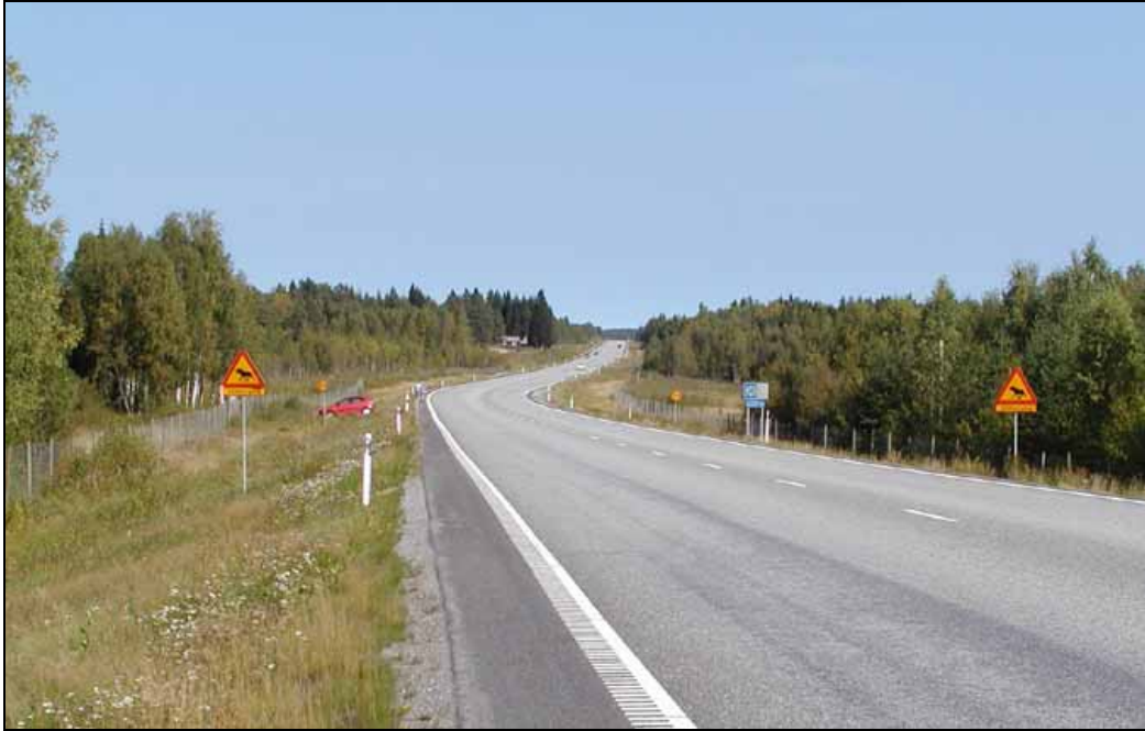
Figure 4.11: Warning signs in Rosvik, Sweden (Photo: Andreas Seiler)
