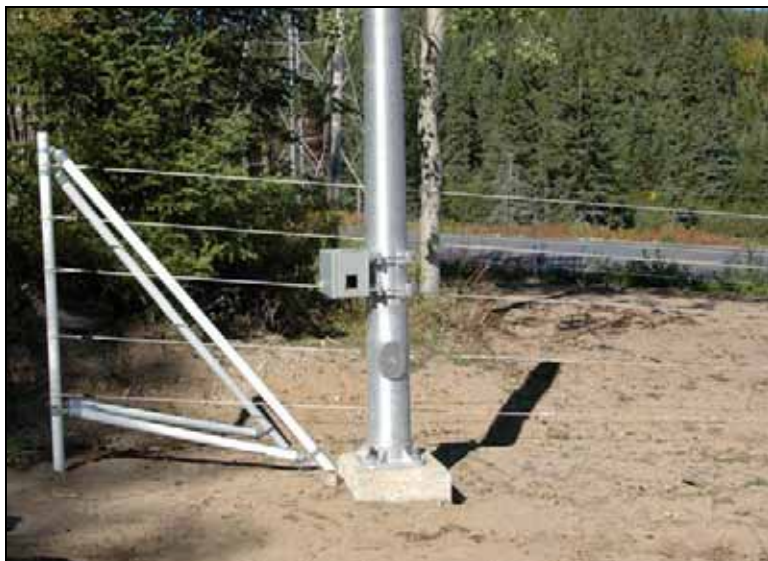
Figure 4.41: Sensor and electric fence in Herbertville, Quebec, Canada (Photo: Ministère des Transports du Québec)
