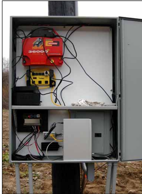
Figure 4.42: Control cabinet in Herbertville, Quebec, Canada. The upper section of the control cabinet contains the electronics for the electric fence; the lower section contains the electronics for the sensors and warning signals. (Photo: Ministère des Transports du Québec)
