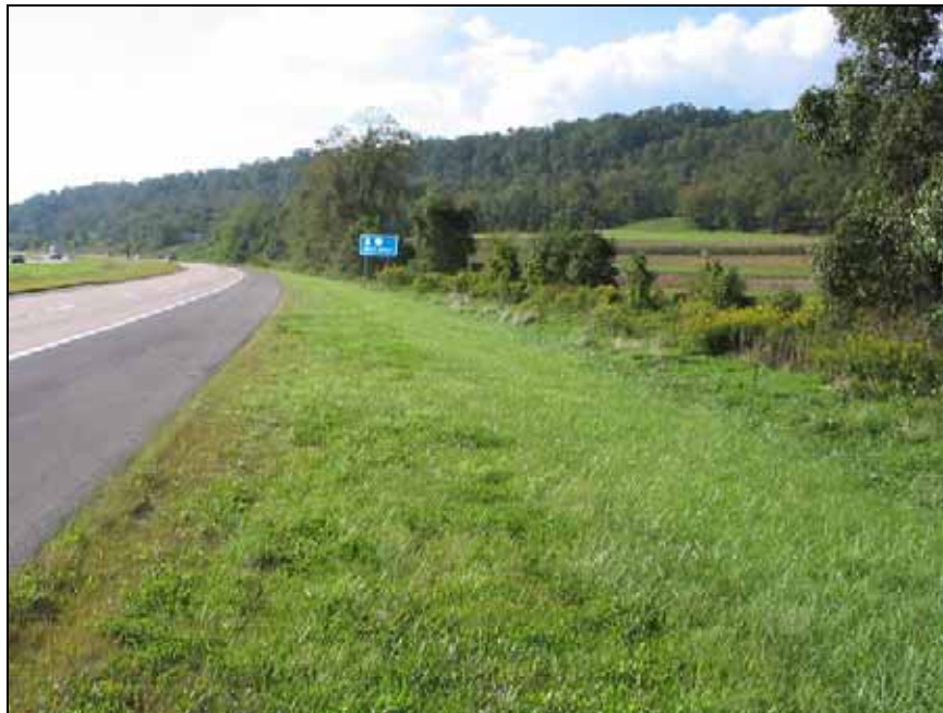
Figure 5.5: View of Westbound Lanes Hwy 22/322, Thompsettown, PA (Photo: Marcel Huijser, WTI-MSU)
