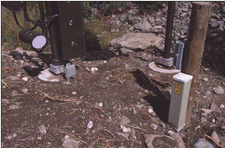
Figure 8.2: The problem with some of the concrete foundations was addressed by putting weed free soil around the posts while not blocking the drainage from the road. (Photo: Marcel Huijser, WTI-MSU)
